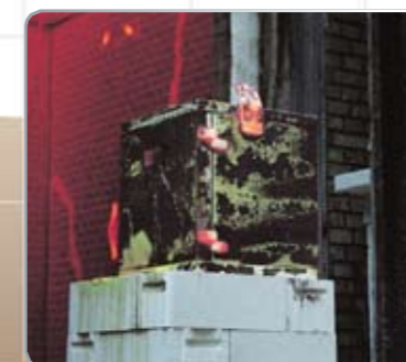
Removal of cabinet from oven
